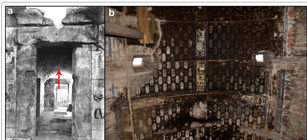
Fig. 2 a Black and white photograph from 1930s of the sanctuary of Osiris (looking to the West), showing the vaulted ceiling covered with black soot layers (red arrow) [13]. b Photograph of the painted ceiling of the sanctuary of Osiris, largely covered with soot
